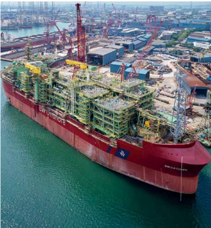
Keppel Shipyard is on track to deliver its twelfth FPSO, BW Catcher, to BW Offshore. Upon its completion, BW Catcher will be deployed to the Catcher Field located in Central North Sea, UK
