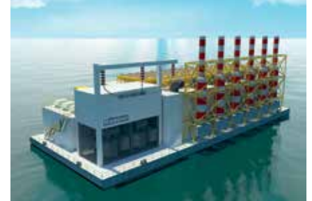
Keppel's Floating Storage and Regasification Power Plant (FSRP) integrates the storage and regasification units to provide efficient LNG power generation in a single economic package
